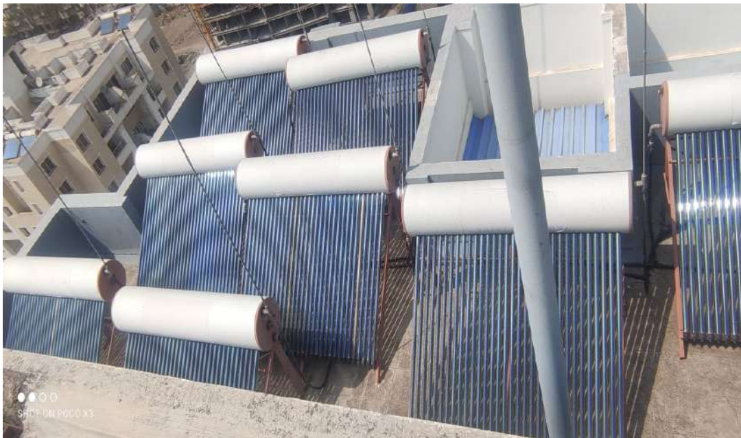
SOLAR HOT WATER PANELS
