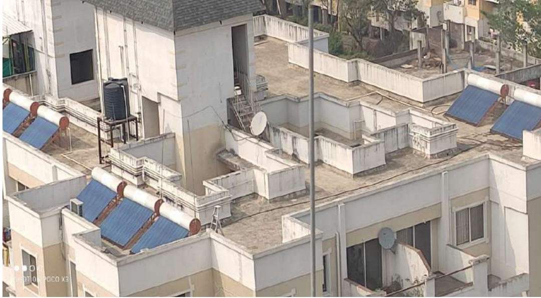
SOLAR HOT WATER PANELS
